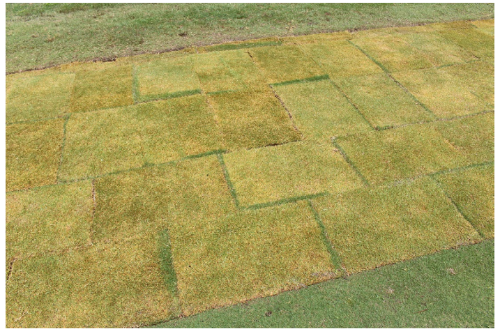
Figure 2. Correctly staggered sod seams. Notice that this sod has been on a pallet for several days but will still recover if adequate moisture is applied immediately after laying.
