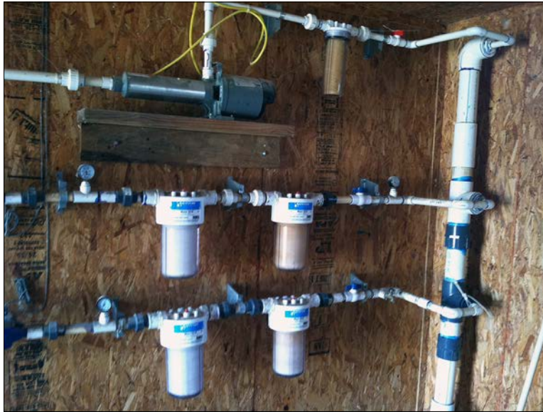
Figure 3. A 4-inch supply line from the well with 1-inch distribution lines to the drinkers in the front and back halves of the house and to the cooling system.
