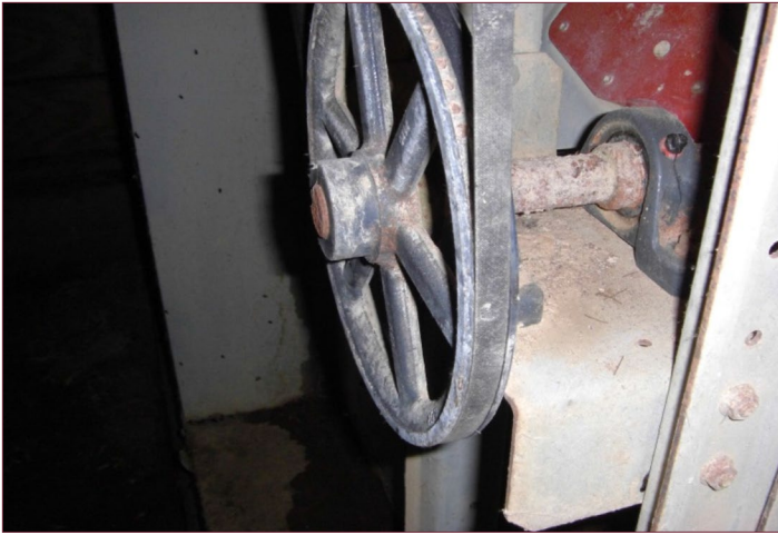
Figure 2. Belt-drive fans have bearings and grease fittings that need grease twice a year.
