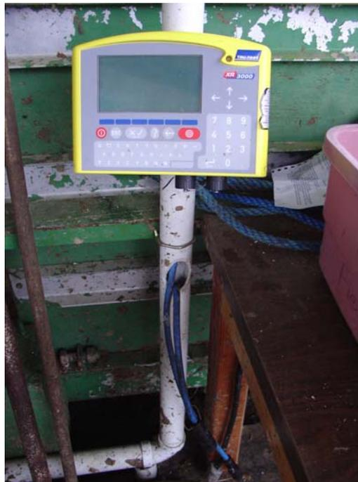
At the South Farm on the Mississippi State University campus, David Pinkerton built a device out of 2-inch PVC pipe to protect the cords running from the load bars of the digital cattle scale to a mount for the digital indicator. The PVC pipe not only protects the cords from damage, but it also keeps them out of the way during cattle working.
