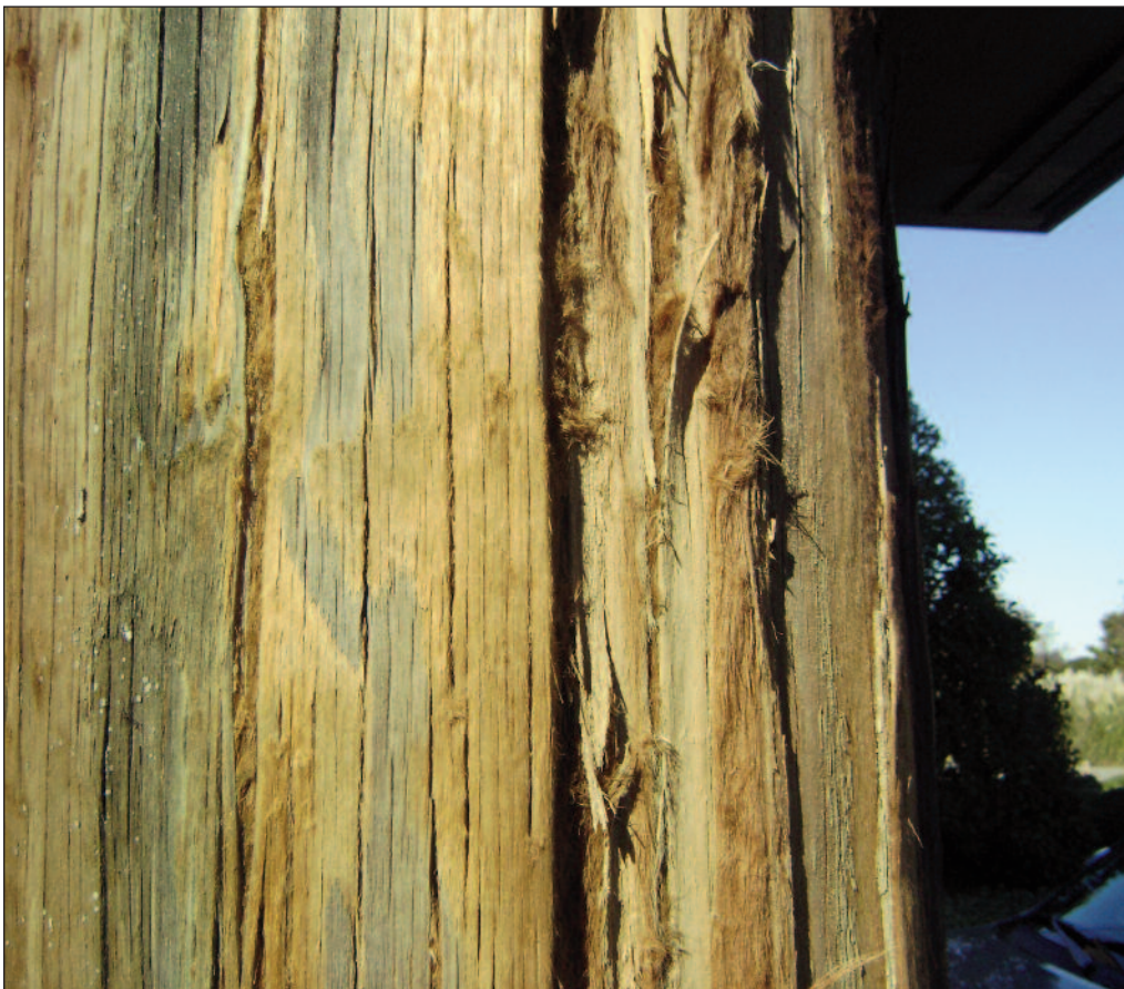
Figure 1. The chlorine in salt can, in certain circumstances, slowly degrade wood. High salt concentrations, high moisture levels, and warm temperatures can accelerate the process.
