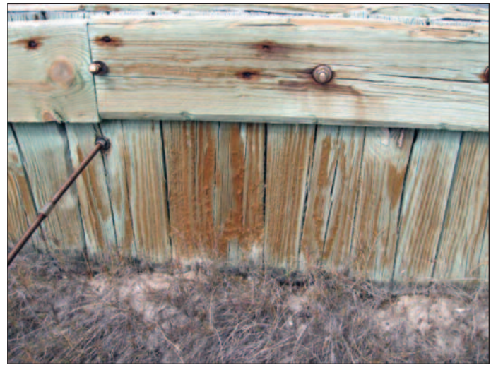
Figure 3. Salt kill occurs as intertidal salt from the water is deposited on the wood structures or wicks upward in the wood.
