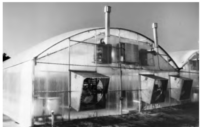
Proper sizing of the exhaust fans is important to ensure adequate temperature control during warm periods. Refer to the text for the simple calculations.
