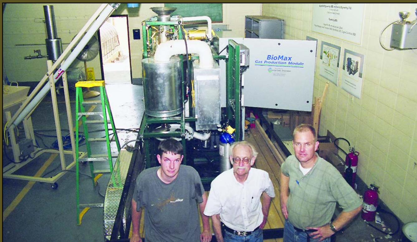
Community Power Corp. technicians Mike Walker, left, Jim Diebold and MAFES agricultural engineer Alex Thomasson during installation of the Biomax gasifier.
